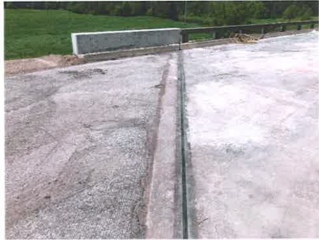
Photo 2: Compression Seal Installed
