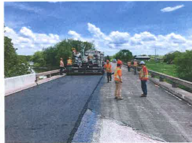
Photo 4: Asphalt Placement
