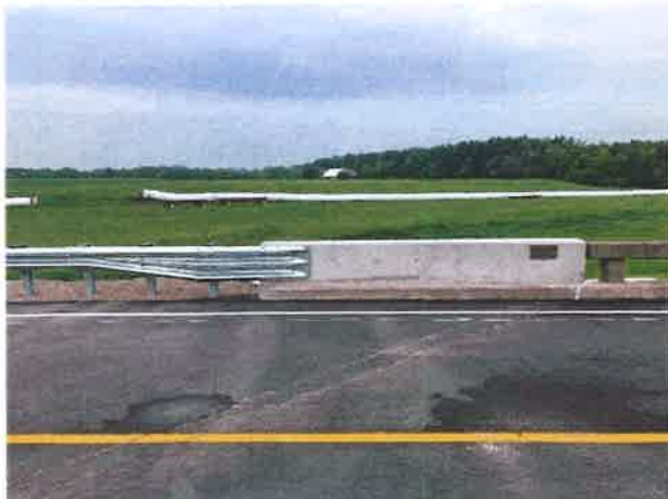
Photo 5: Guide Rail Structure Connection
