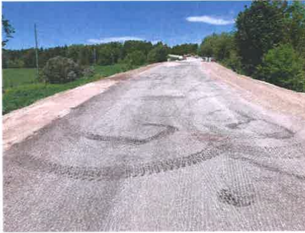
Photo 1: Milled Asphalt on South Approach
