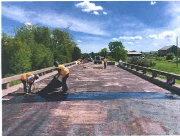
Photo 3: Waterproofing Deck Top
